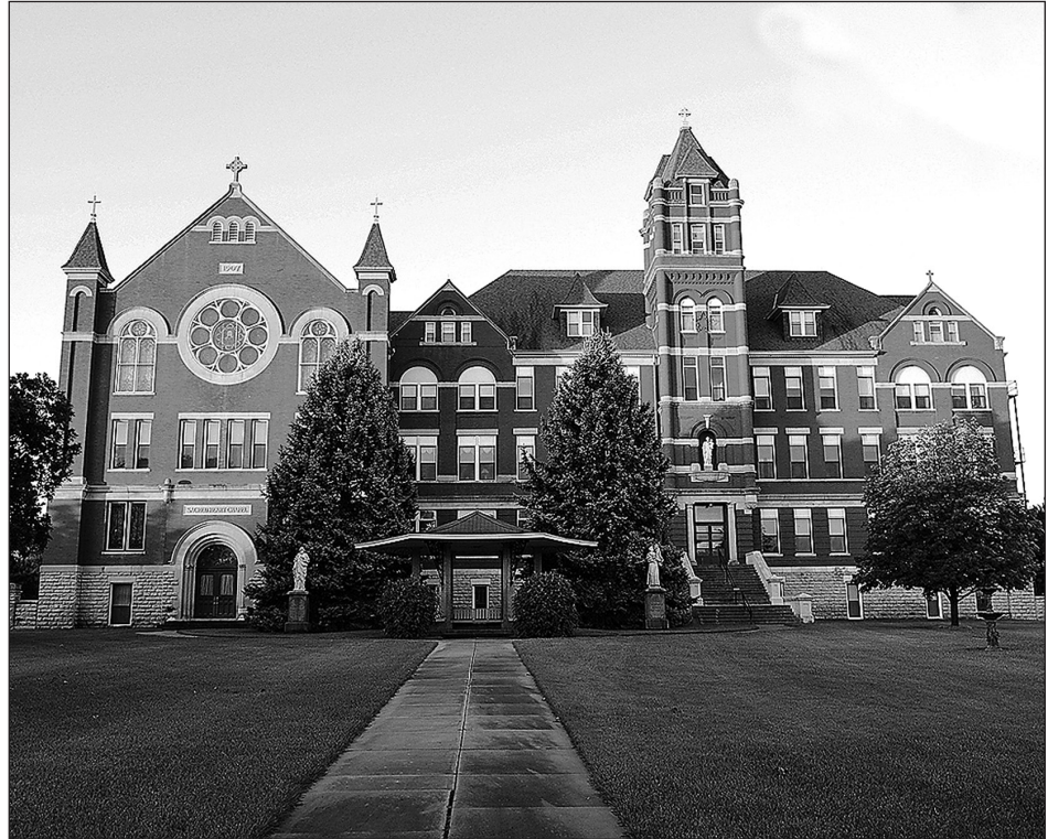
The Nazareth Motherhouse in Concordia has a lot of square feet of roof to replace. Does this remind you of Marymount?
